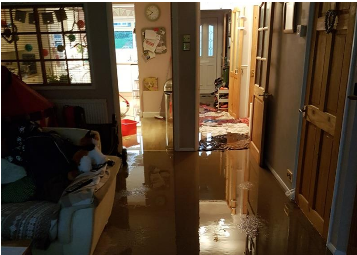
Photograph 3: Internal property flooding
