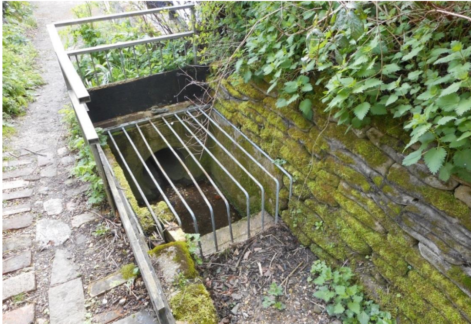
Photograph 6: A culvert on a small watercourse
