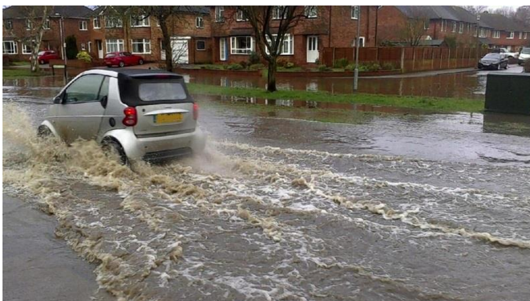
Photograph 1: Floodwater affecting the highway
