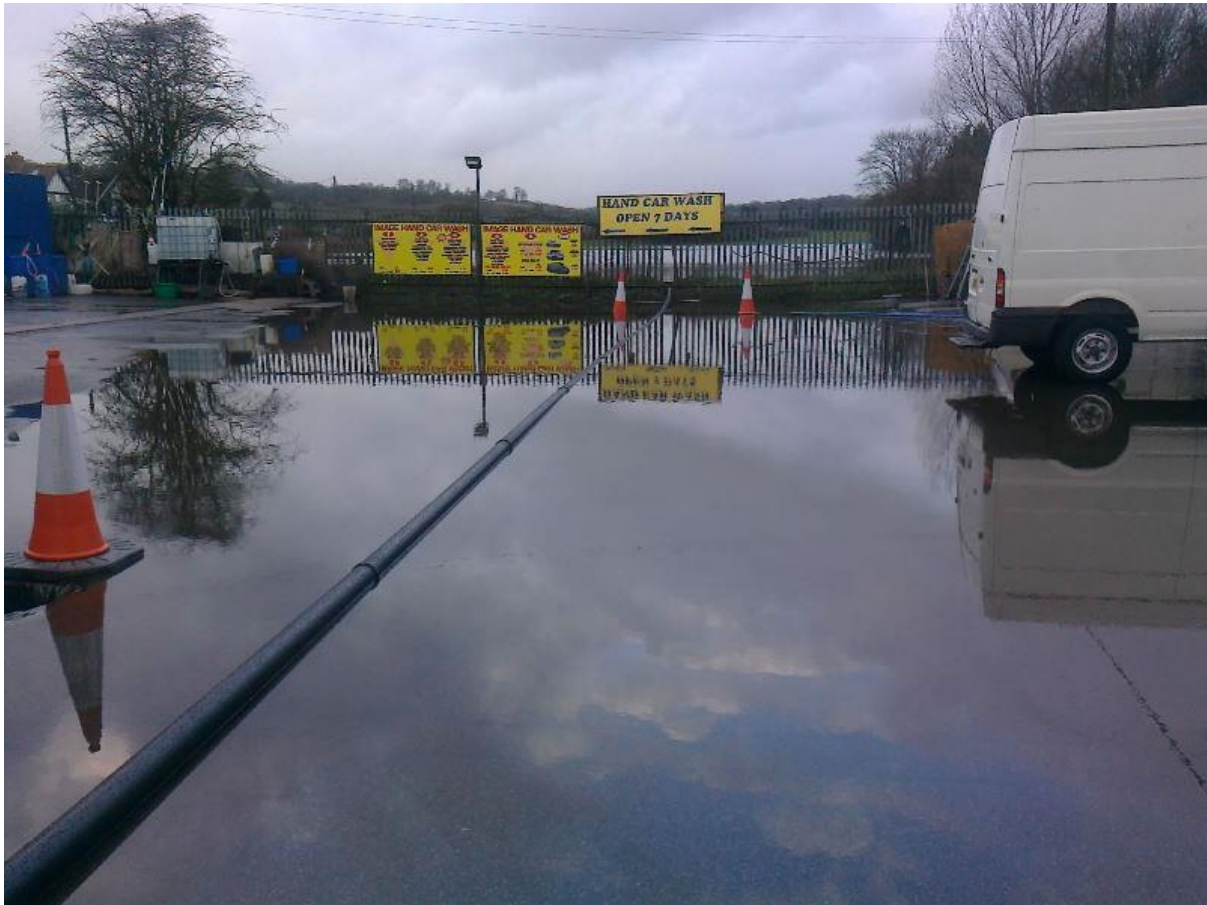
Photograph 10: Extensive groundwater flooding
