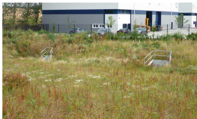
SuDS attenuation basin, Bourne End, Dacorum
