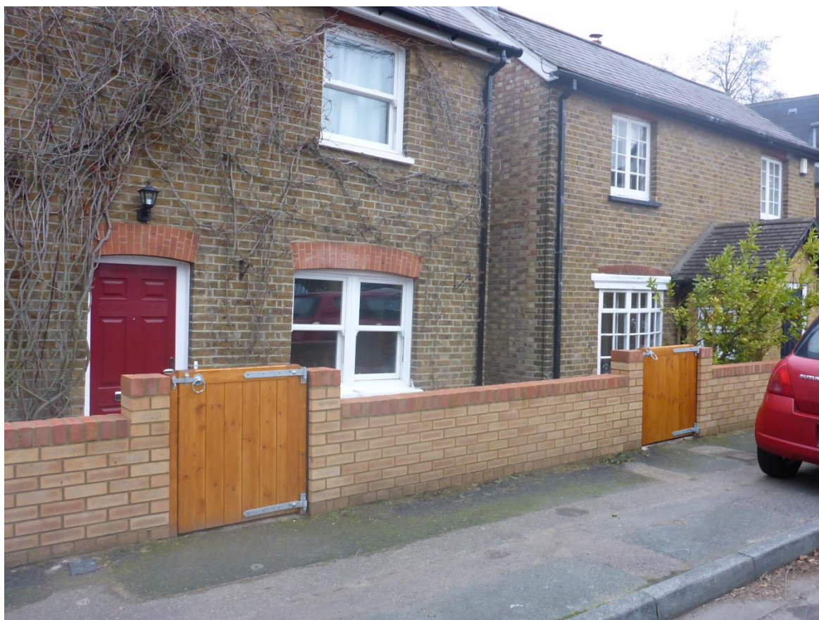
Photograph 18: Boundary wall and flood gates
