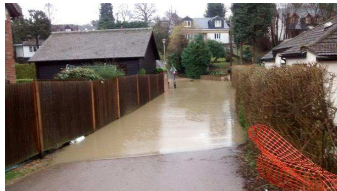
Flooding in Robbery Bottom Lane, Welwyn
